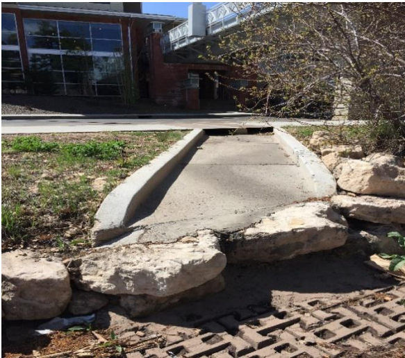
Figure 7: "Open Inlet" After Pedestrian Bridge on McConnell Drive
