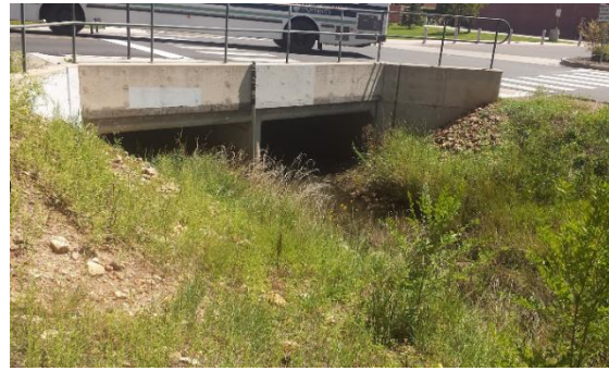
Figure 3: DBC Crossing Under Knoles Drive [3]
